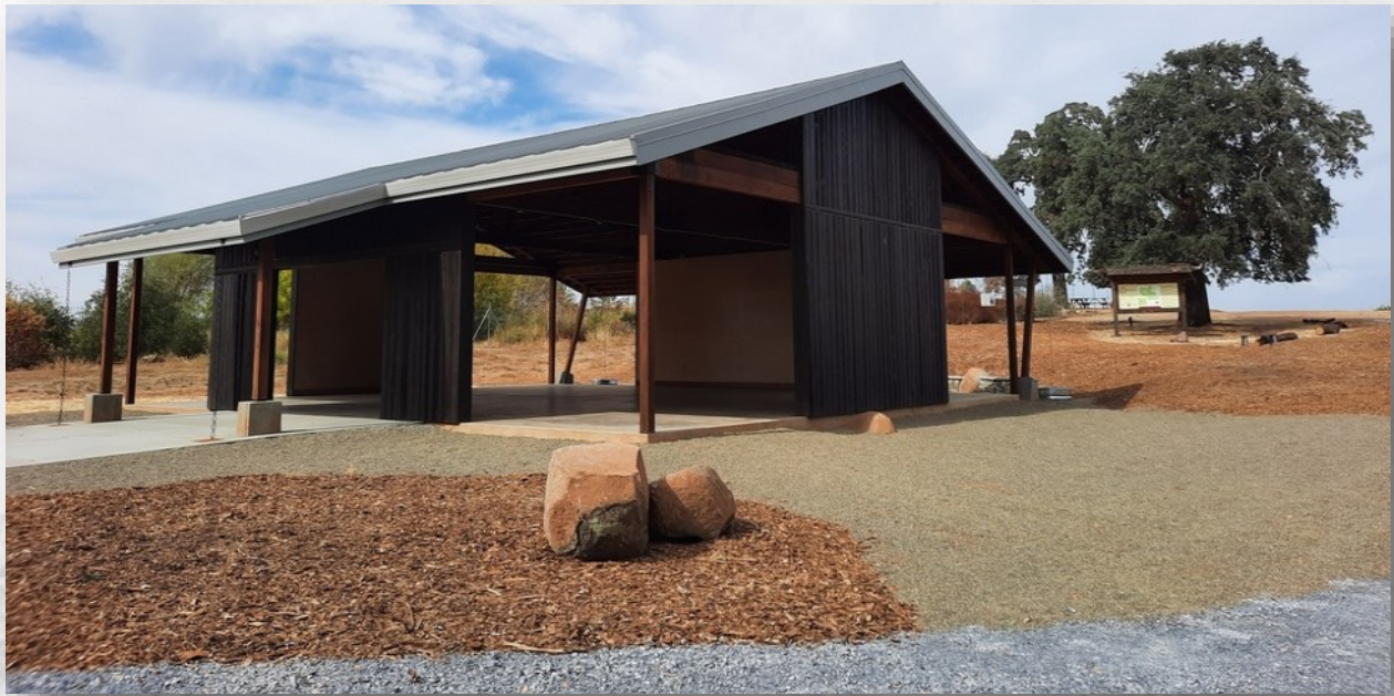
Phase 1 of ARC's new Education Center - now complete!
